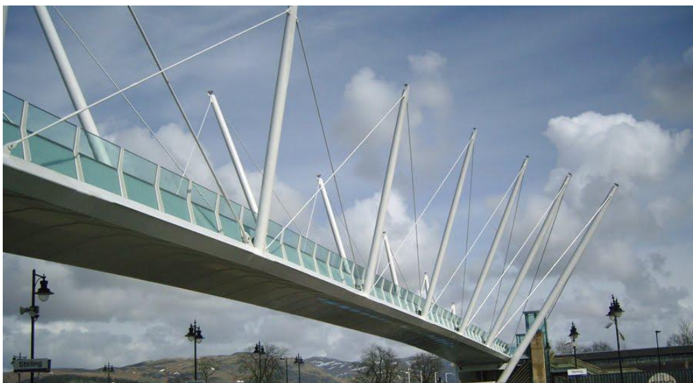
Fot.27. Forthside Bridge, widok z boku [37]
